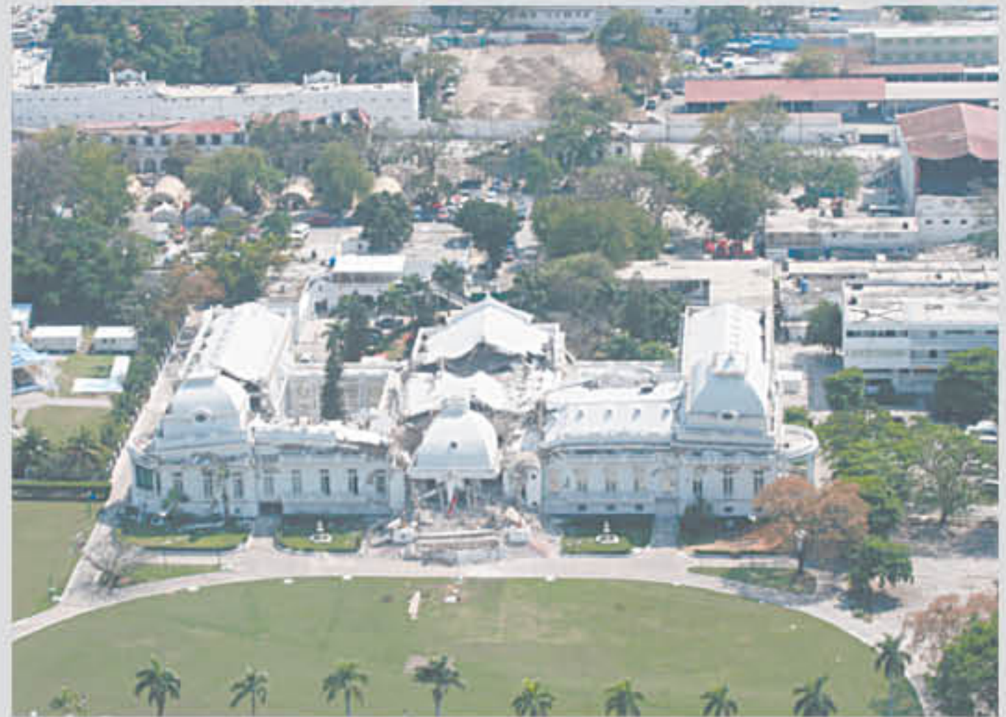
The Haitian Presidential Palace Post The 12 January 2010 7.0 Magnitude Earthquake
