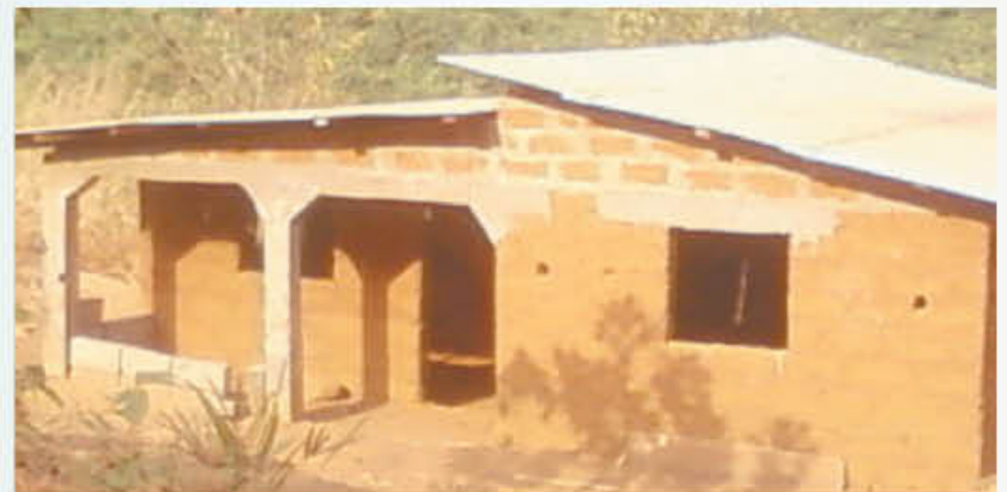
One of the many houses in Sierra Leone made from mud and concrete blocks.
